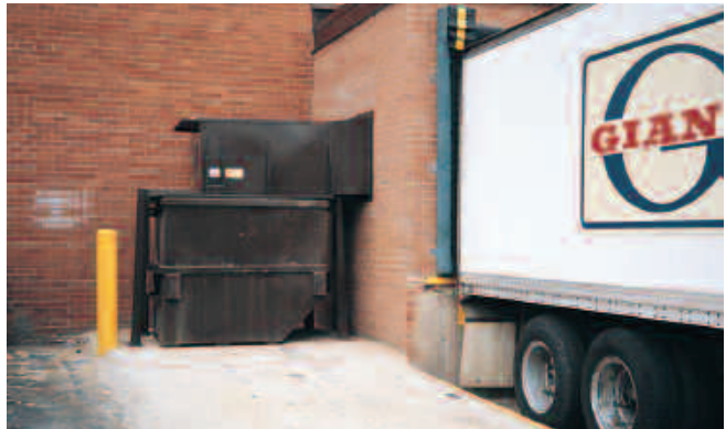
Installed at a supermarket, this side feed VIP is equipped with an optional "thru-the-wall" security chute enabling the unit to be fed from inside the building. The security chute controls employee pilferage by eliminating the temptation to put merchandise into a box, stash the box in a trash container and return at night to retrieve the merchandise. The refuse is totally enclosed with no access to scavengers – or children who play on or in anything available!
